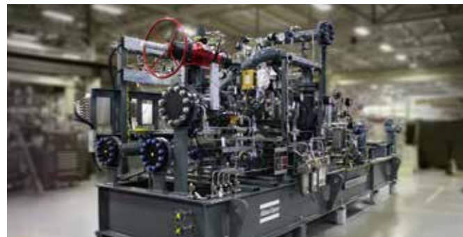
An Atlas Copco fuel gas booster
