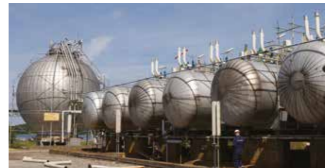
Inside an ethylene-oxide plant
